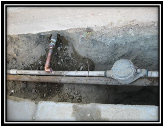
Left: Service pipeline with meter.
