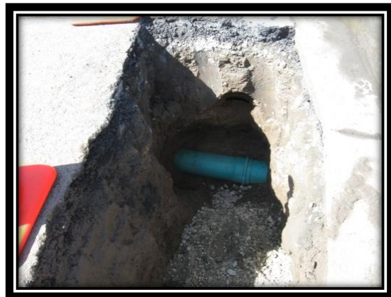
Replacing drainage pipe from new catch basin to storm drain on Golden Triangle Road.
