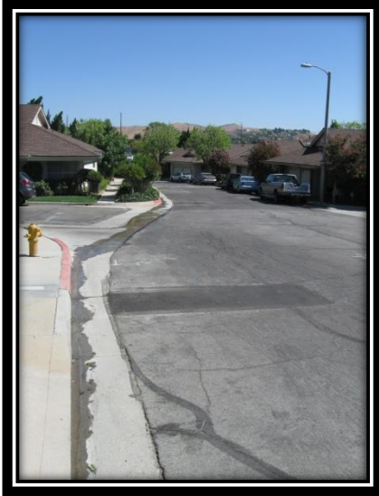
Completed street with patches from service replacement trench work.
