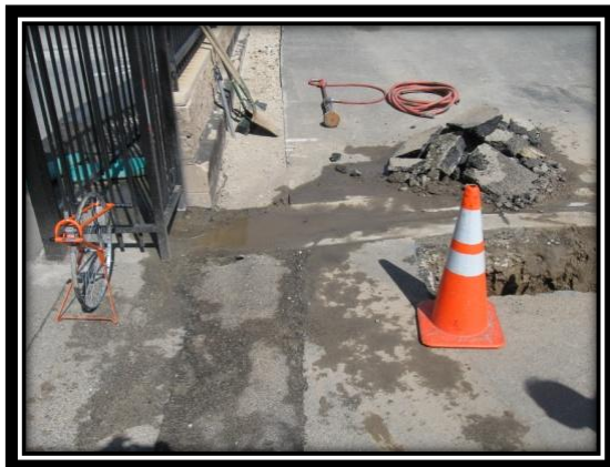
Replacing drainage pipe from new catch basin to storm drain on Golden Triangle Road.
