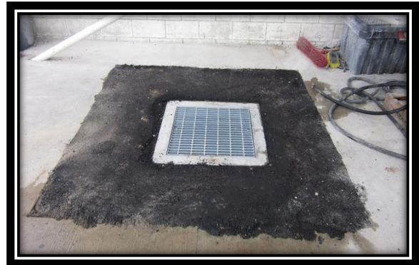
Installing new catch basin south of existing building for better drainage.
