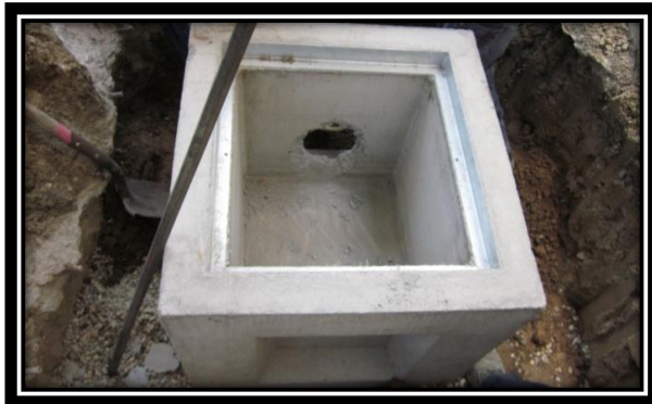
Installing new catch basin south of existing building for better drainage.
