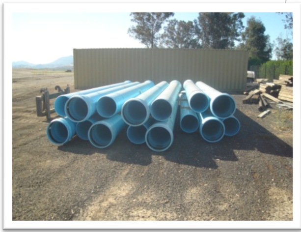
2009 - Agency begins construction of the Rio Vista Water Treatment Plant expansion.
