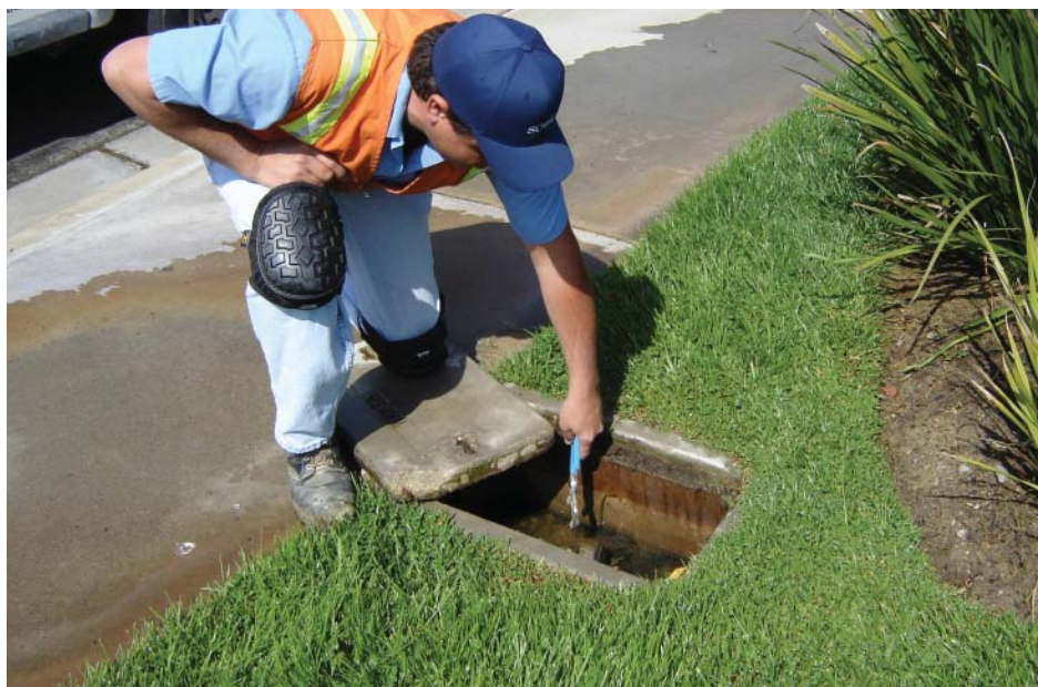
A Division employee conducts routine maintenance.
