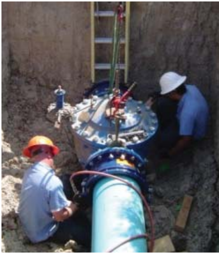
Field crews install an altitude valve at Honby South tank site.
